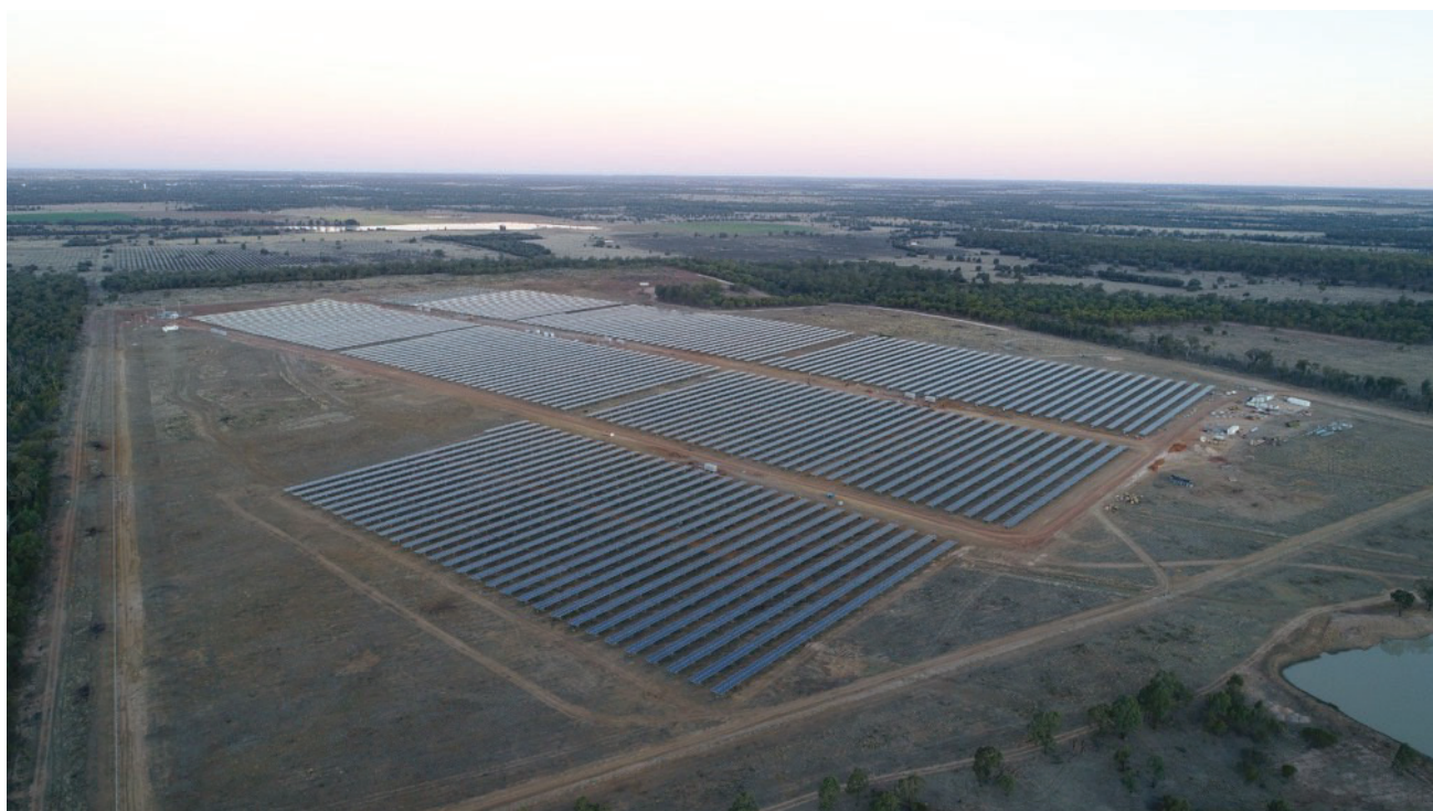
Chinchilla Solar Farm under construction, August 2018.
