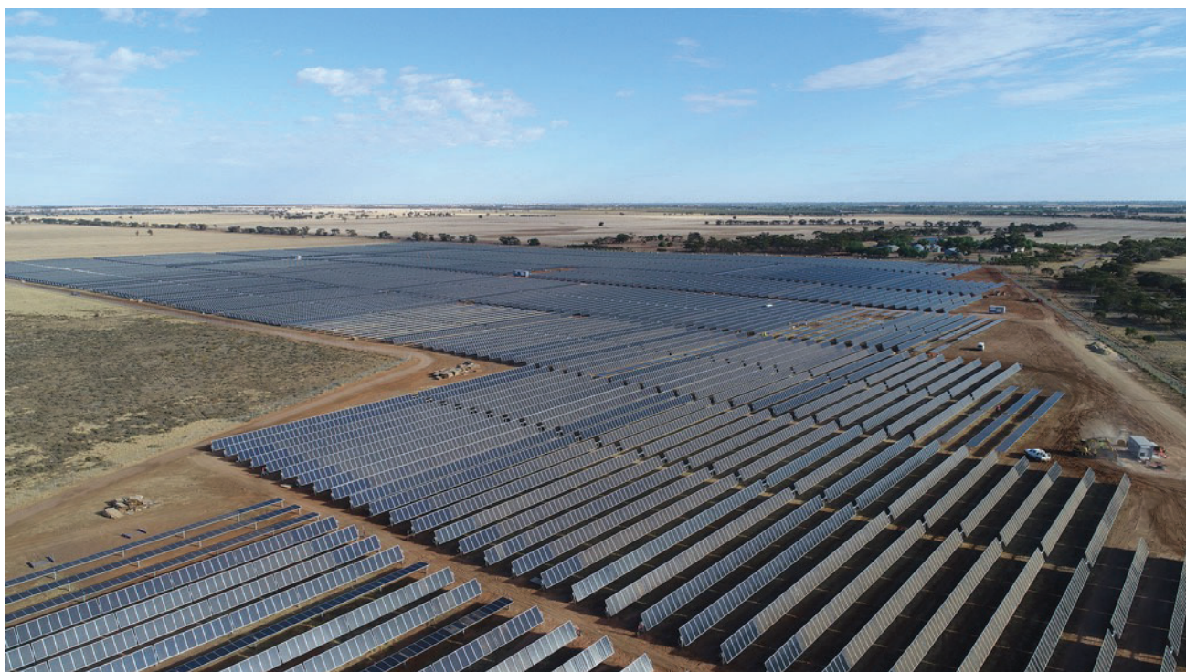
Swan Hill Solar Farm, Panels Complete, April 2018 - Image Courtesy RCR
